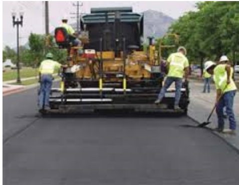
Fig. 3: Laying of EKO-MIX mixture [5].
