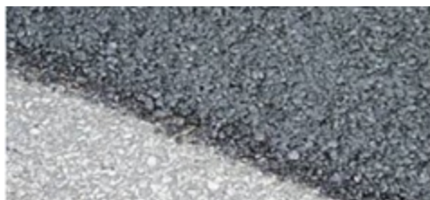
Fig. 8: Very Thin Layer Asphalt Concrete [17].
