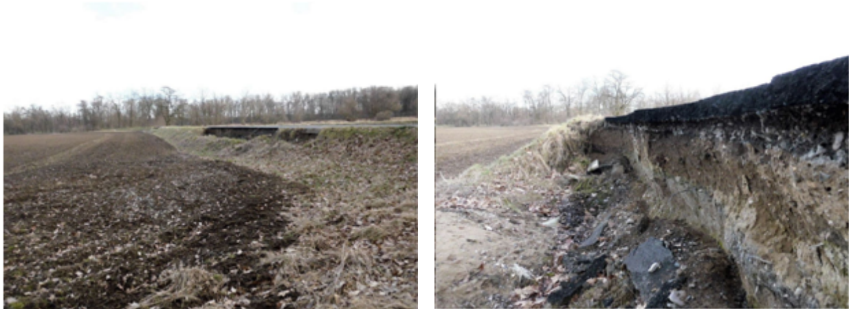
(a) the greatest of the many failures of downstream face of the levees in the length of approximately 25 m
