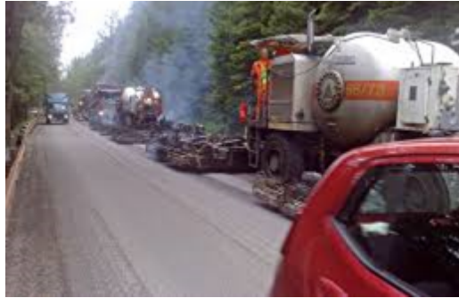
Fig. 5: Construction of new pavement with recycling machine by cold technology [14].
