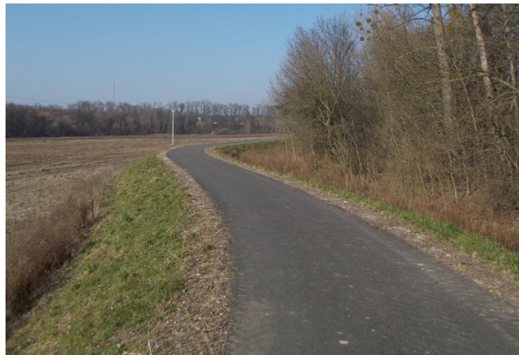
Fig. 2: Levee with asphalt bicycle trail near the village Rohatec in the Hodonín ( http://standa1977.rajce.idnes.cz ).
