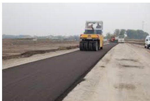
Fig. 2: Production and laying of Valorcol technology [4].
