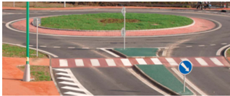
Fig. 1: Laying of Végécol technology in Myjava [3].
