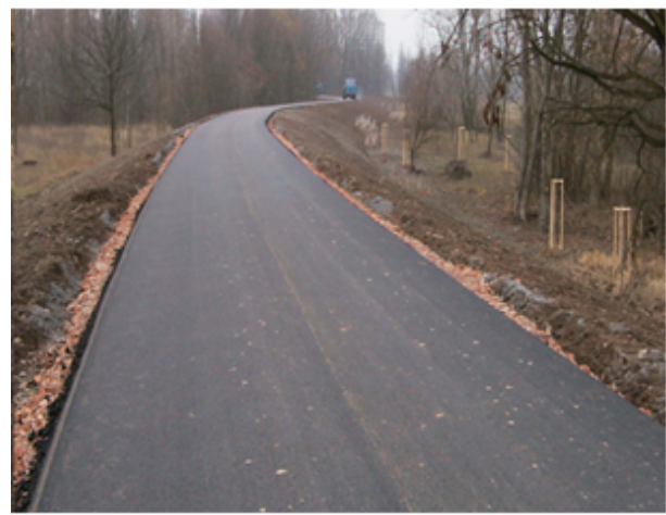
(b) levee after construction
