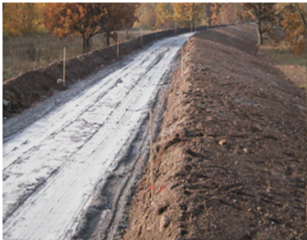
(a) levee during construction
