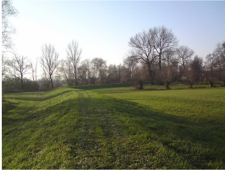
Fig. 3: Completed levee near the village Nepasice ( http://reka-orlice.sije.cz/trebechovice-hradec-kralove ).
