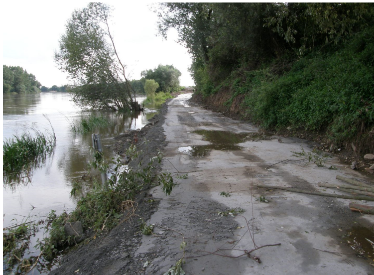
Fig. 8: Flooding of base layer of still unfinished cycle paths from CCB during flooding (ČEZ a.s., 2013).
