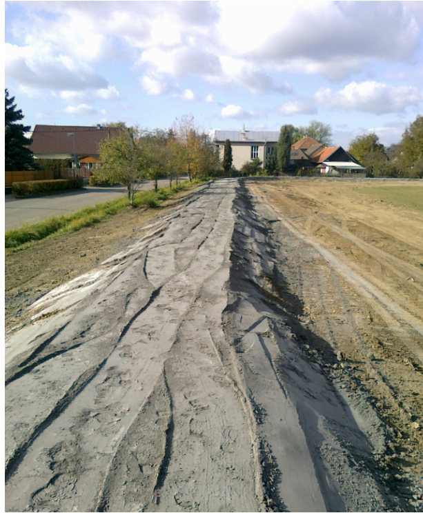
Fig. 5: Vrды - construction of levee using CCB (Power Plant Opatovice, 2014).
